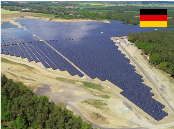
SolarTerrace MAC Germany 63MW
